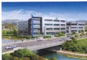
Australian Office Eastside Building - Robina
